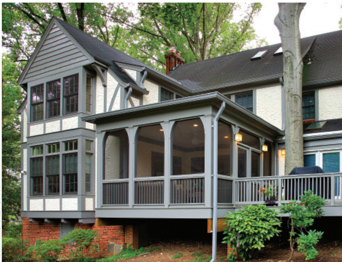
PHOTOGRAPH COURTESY OF: GILDAY RENOVATIONS
